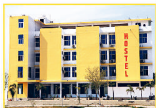
AC Hostel Facility For Boys & Girls
